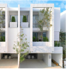
THE RESIDENCE BY ANDAMAN ASSET SOLUTION
